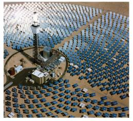
Figure 6. A Department of Energy-sponsored pilot solar thermal project built in California's Mojave Desert in 1981, shown here, was a 10-megawatt power tower surrounded by more than 1,800 sun-tracking mirrors [12]
