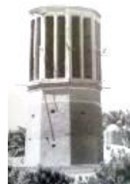
Figure 5. Small garden in body of the wind catcher for evaporative cooling [16]
