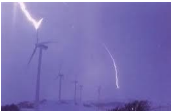
Figure 1(d). An example of lightning damage
