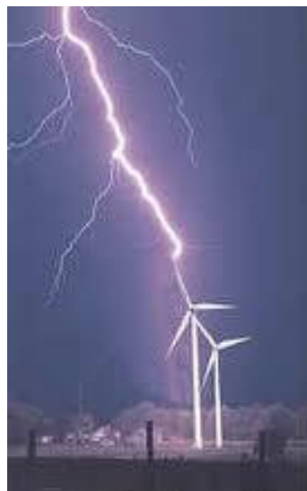
Figure 1(a). An examples of lightning damage
