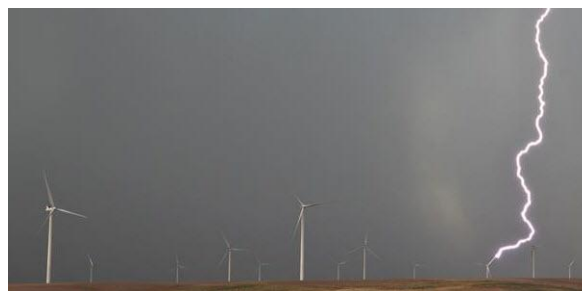
Figure 1(c). An examples of lightning damage
