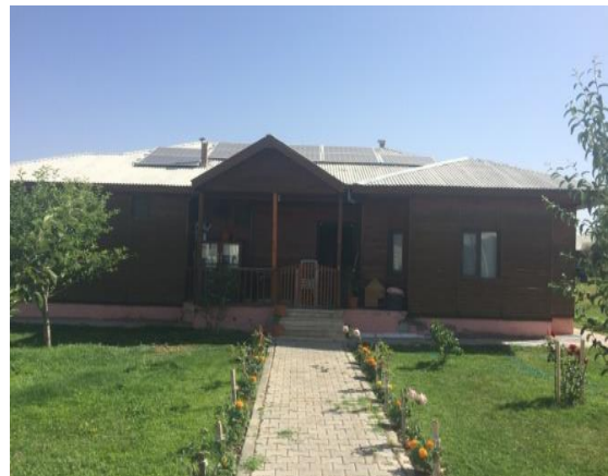
Figure 6. The array of PV panels
