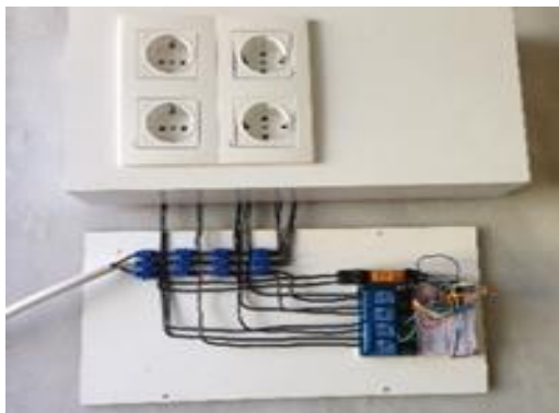
Figure 10. The mounted hardware structure
