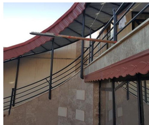
Figure 10. Lighting of LED passages and installed environment to implement the second scenario
