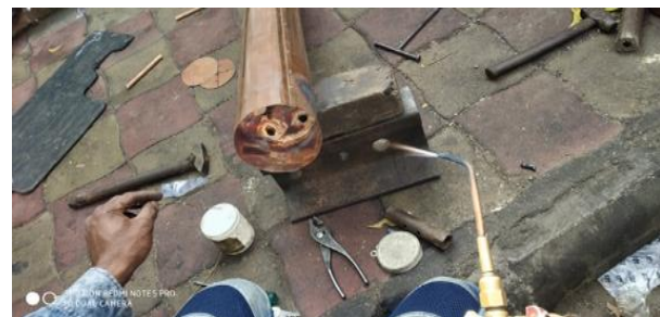
Figure 7. Brazing of tube inside the shell
