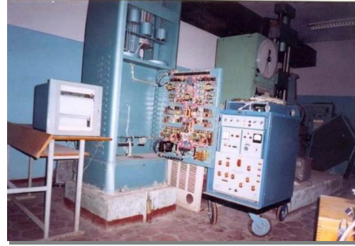
Figure 1. Electrical equipment installation of AIMA-5-2
