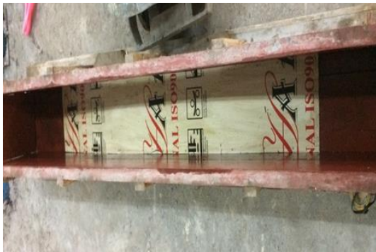
Figure 3. Details of wood molds
