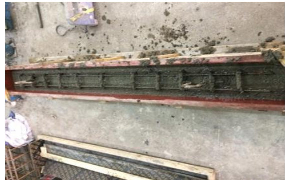
Figure 5. Casting the first layer of mixture
