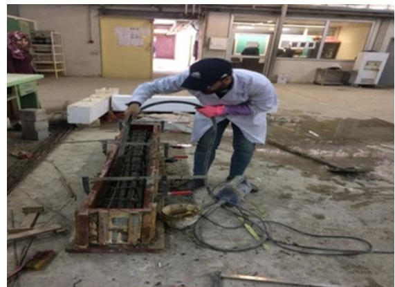
Figure 6. Vibrating the mixture
